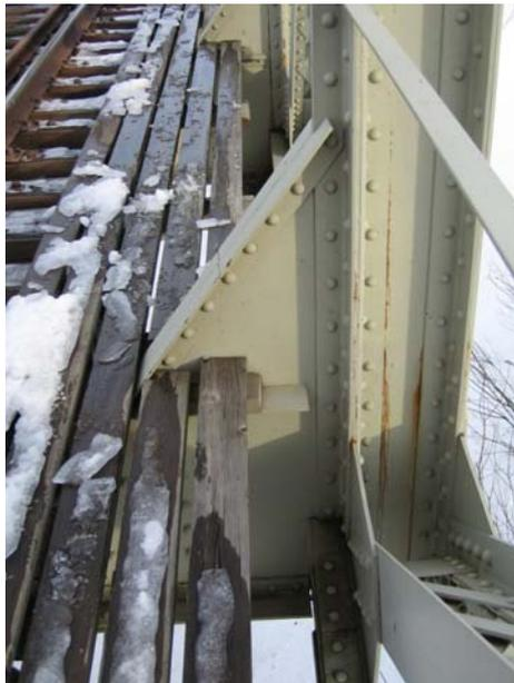
Figure 7.2 Connection between cross girder and the main truss, Enochsson (2007)
