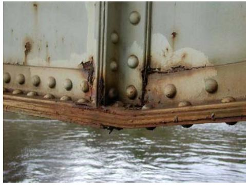
Figure 5.11 Example of corrosion on a plate girder bridge
